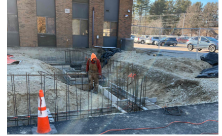
Above: Foundation work at new Science towers.
